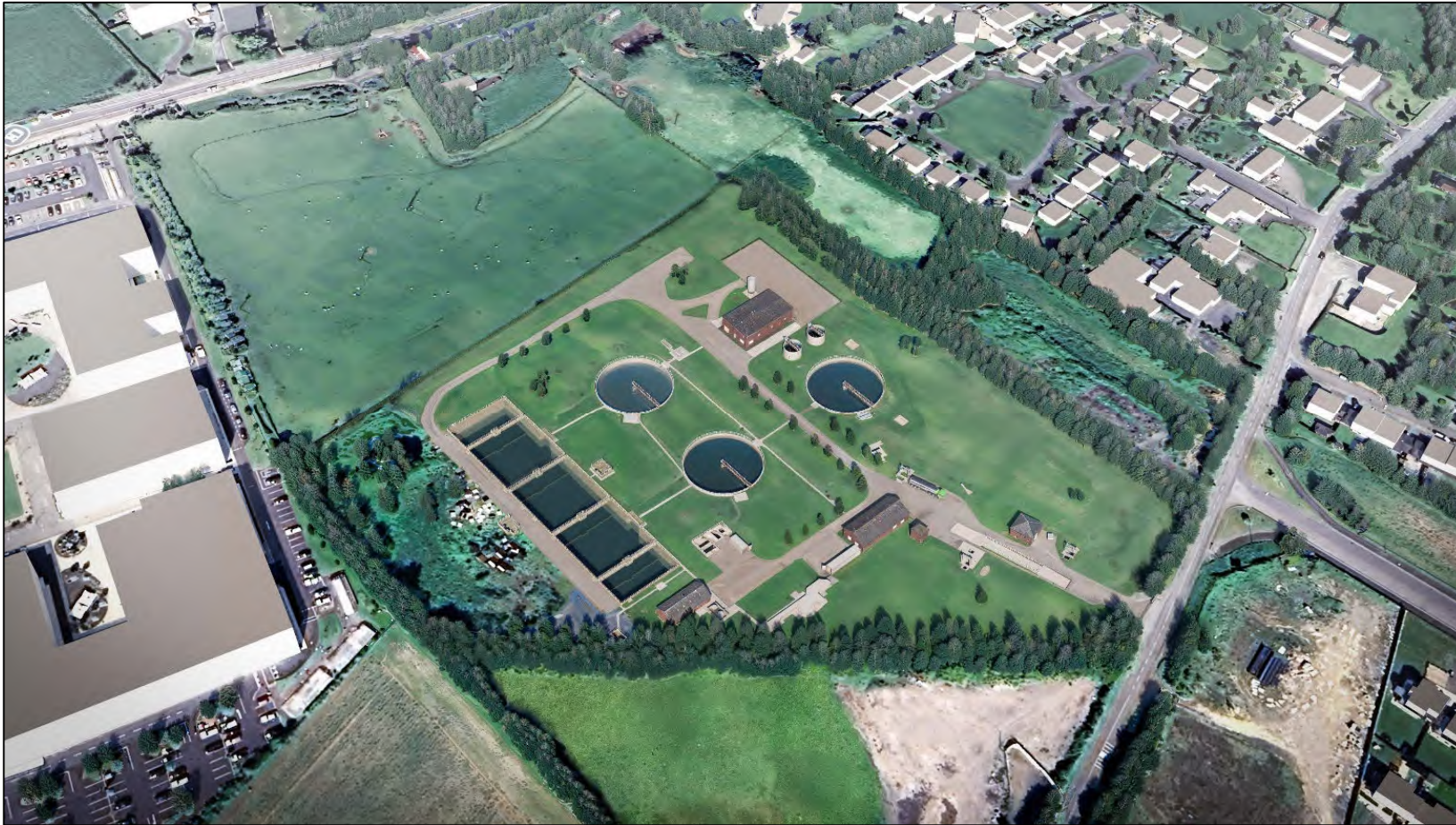
Figure 1-2 – Existing WwTP Site (3D Visualisation) 1
