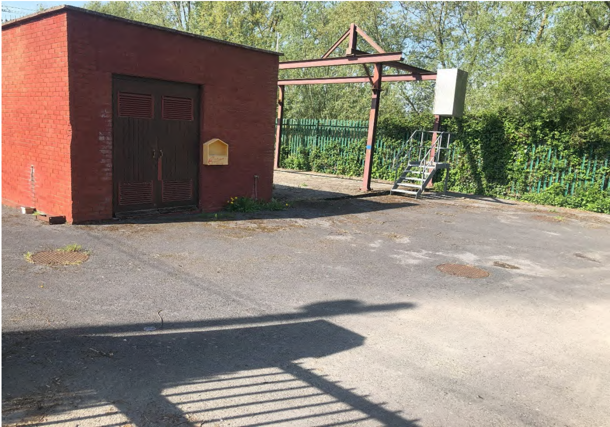
Plate 11-4 Existing Pumping Station
