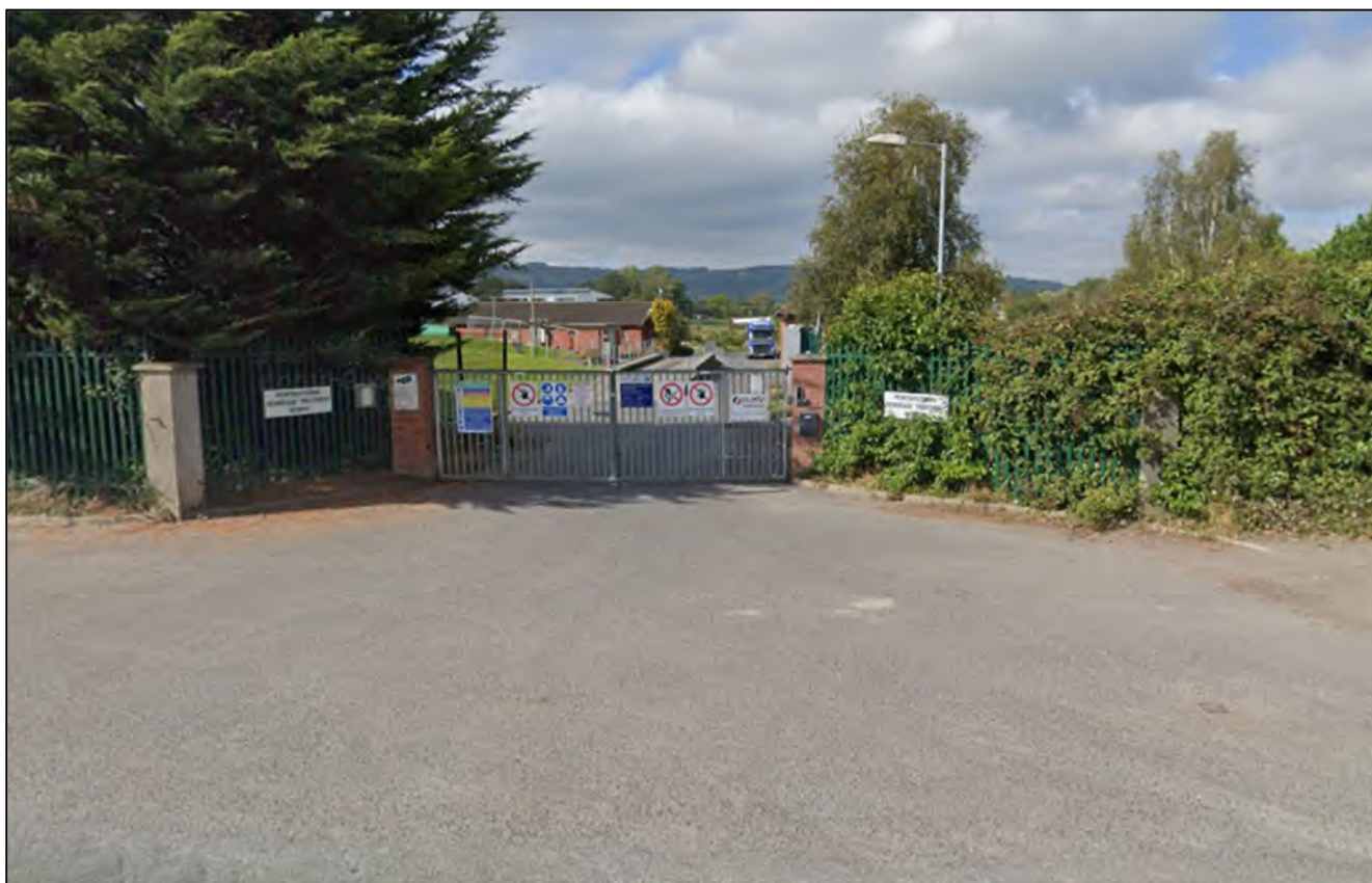
Figure 10-3 - Existing Site Access along Green Road
