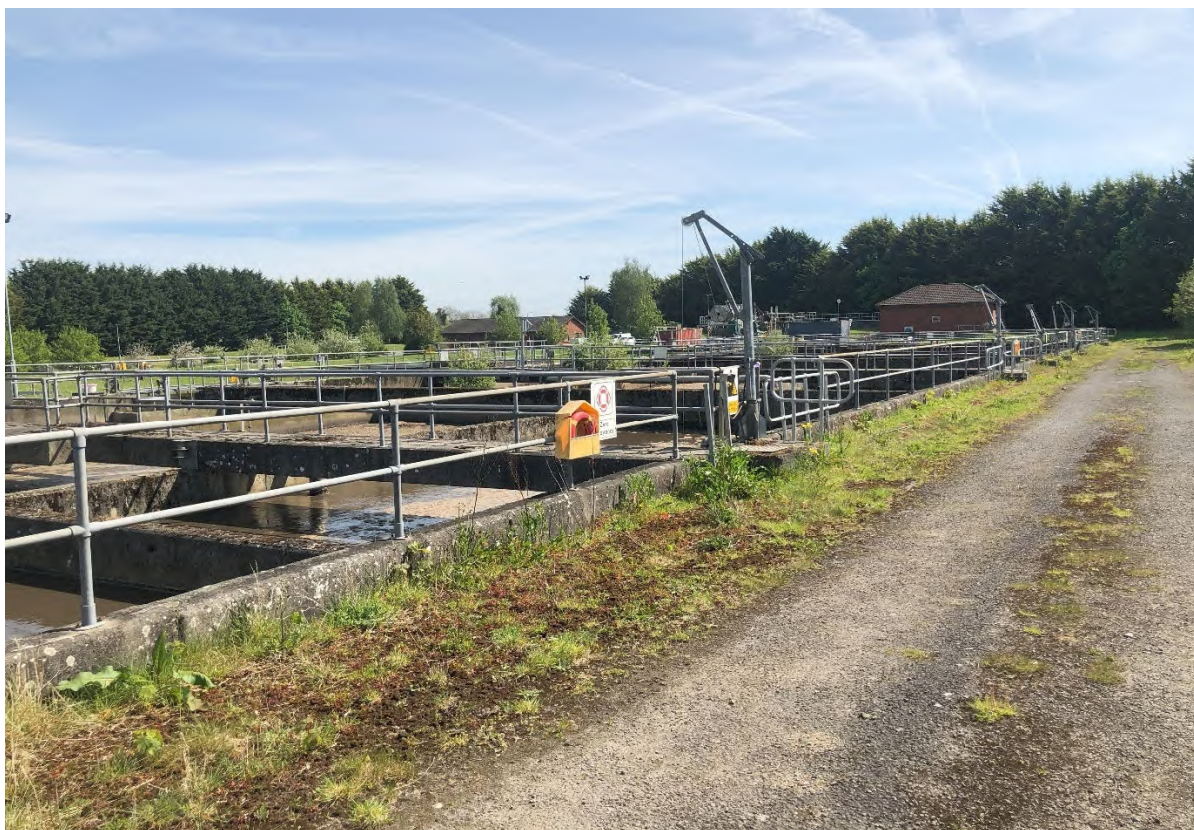
Plate 11-3 View of Waste Water Treatment Plant
