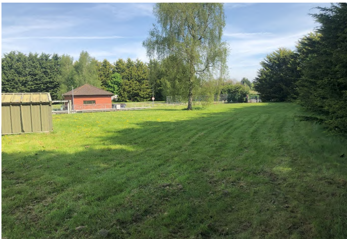
Plate 11-2 Waste Water Treatment Plant
