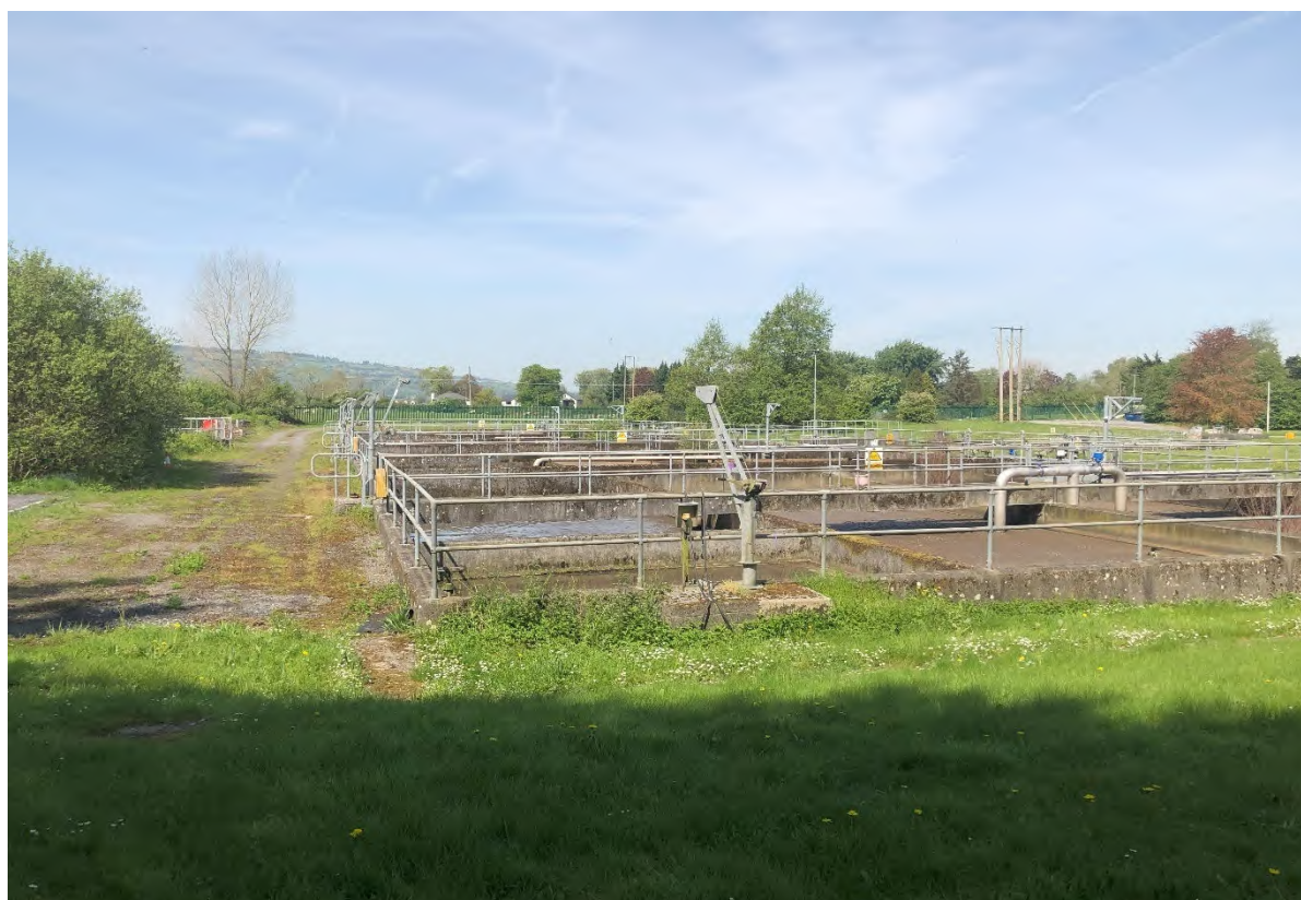
Plate 11-1 Overview of Waste Water Treatment Plant
