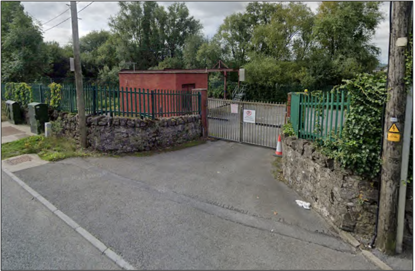
Figure 10-5 – Existing Kilkenny PS Access along Kilkenny Road (R448)
